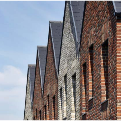
Above – Careful detailing and choice of materials can create distinctive places. St Chad's, Tilbury, Essex
