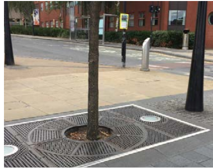
Above – Uncluttered public realm detailing in Sheffield has incorporated lighting adjacent to tree pits and clear pedestrian routes into town
